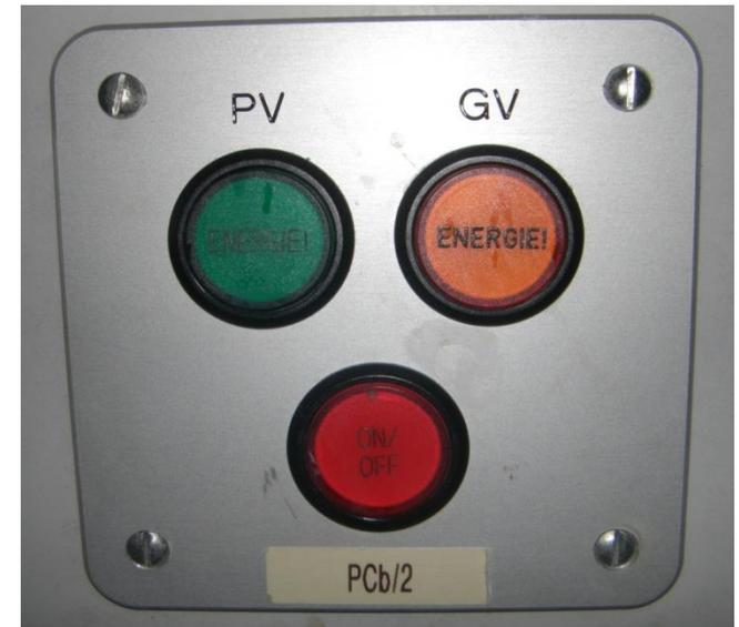
If the **red light** remains on, then the ventilation is **mal-functioning**. Switch the ventilation off and back on, If the problem persists, contact the technical service
